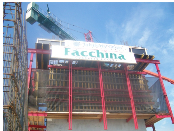
Figure 9.4 – ACS Formwork for Core
